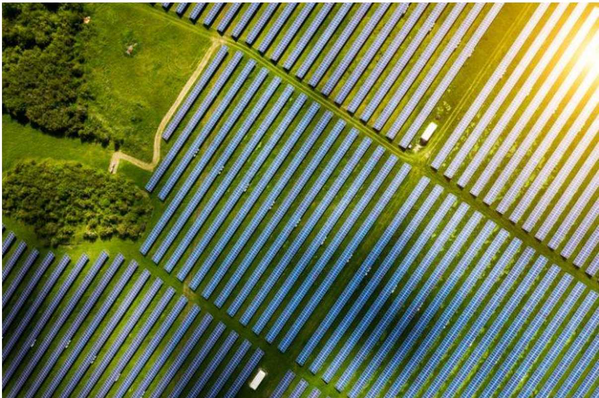
Ground mounted Solar PV showing c 50% land coverage
