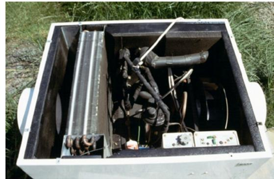
Whilst the heat pump is running, water is continually circulated between the unit and the thermal store by use of a ‘Grundfos’ pump. All piping between the heatpump and store is well-insulated with tight polythene foam insulation.
