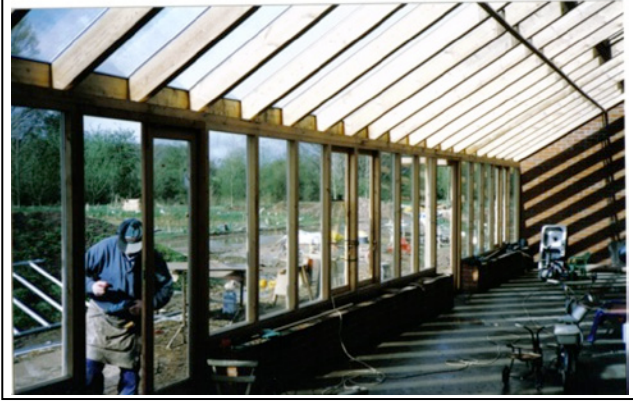
Conservatory glass being fitted
