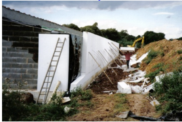
Back wall insulation – Note dpm under insulation
