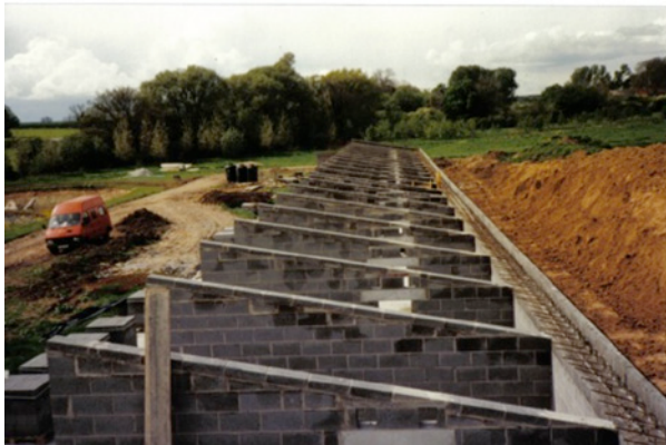
Internal walls making 31 bays
