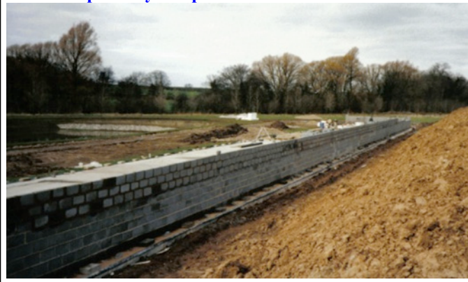
Rear wall partially complete
