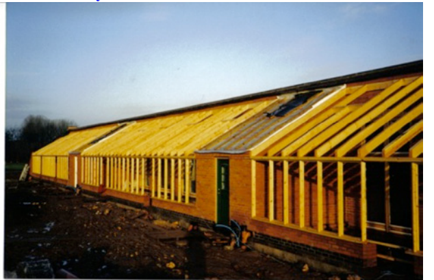
Conservatory timber frame
