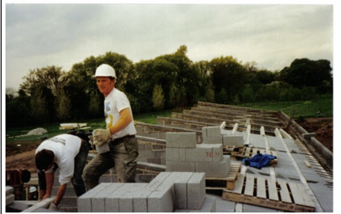
Beam and block roof partially constructed
