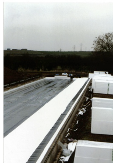
Water proof membrane on blinding slab with insulation placed on top
