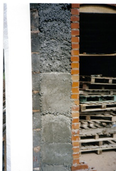
End wall construction showing different layers of materials used
