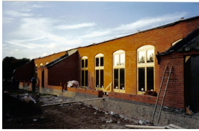
Newly fitted doors and windows to main part of home
