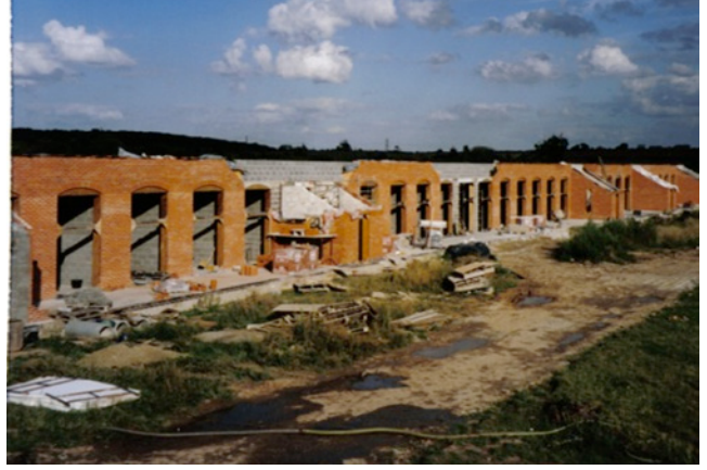
Front wall construction
