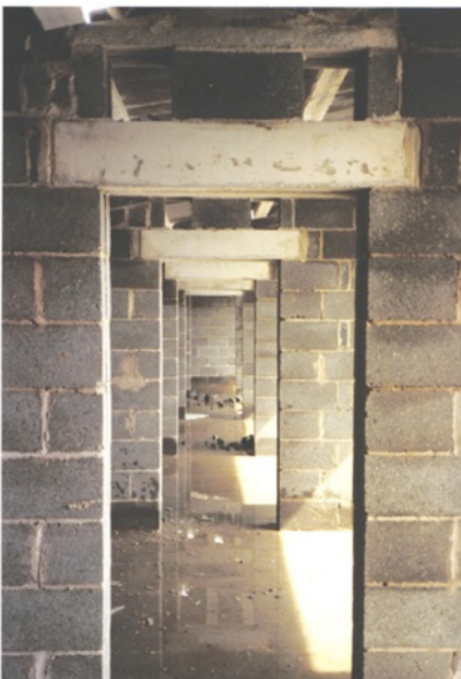
Lintels and provision for ventilation pipes
