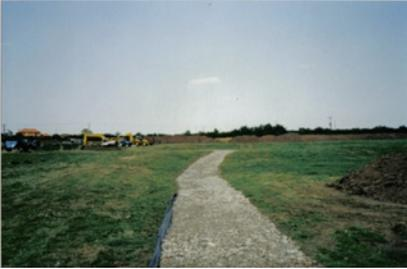
Surface drainage swales were cut along the west side of the roadway, down the east side of the site and across the slope of the site 15m beyond the back wall of the houses. This protected the area of work on the houses from excess surface water, and later formed part of the water drainage/collection system for the non-potable water supply for the homes.
