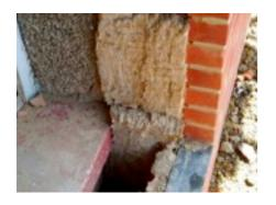
This weakness has been turned into a strength by building an external brick wall, and insulating the resultant cavity between the brick and concrete walls. The original concrete wall will then act as a thermal store, releasing the heat back into the house when temperatures drop.
