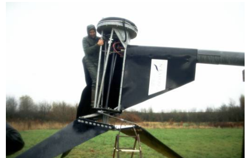
Close up of wind turbine during maintenance work by HHP member
